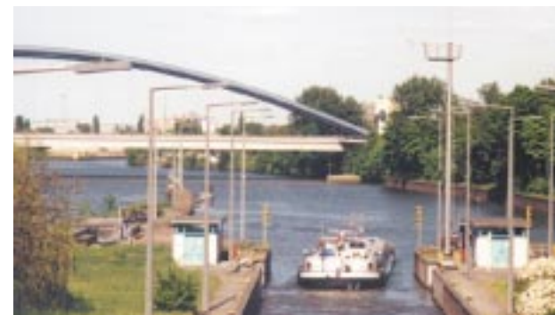
The lock on the River Main at Offenbach.
