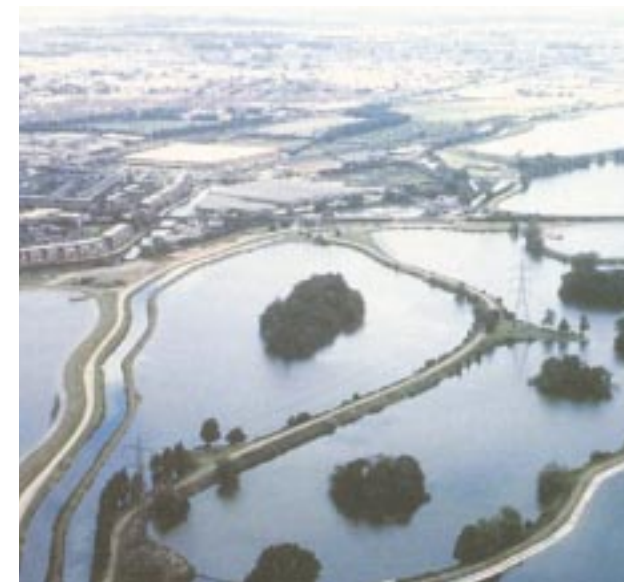
Water Reservoirs in the Lee Valley, East London.
