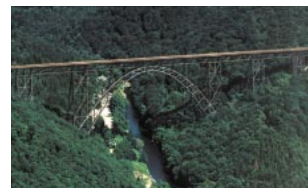
The highest railway bridge in Germany – Müngstener Bridge.
