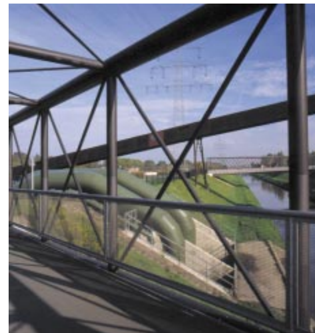
The canalised Emscher in the industrial landscape.
