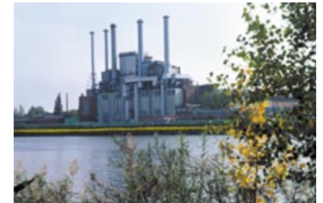
Opel power station, Rüsselsheim.
